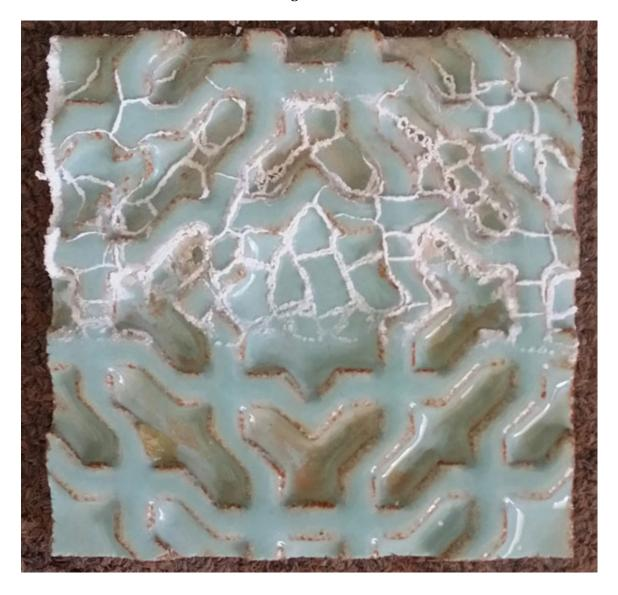
In this case simply wiping the tile down was ample to clean the efflorescence off.
